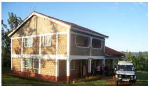
The project building in Kenya at the heart of the comprehensive spread of the VCA.
